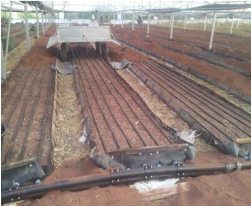
Embedded heating pipes in root zone during soil covering
