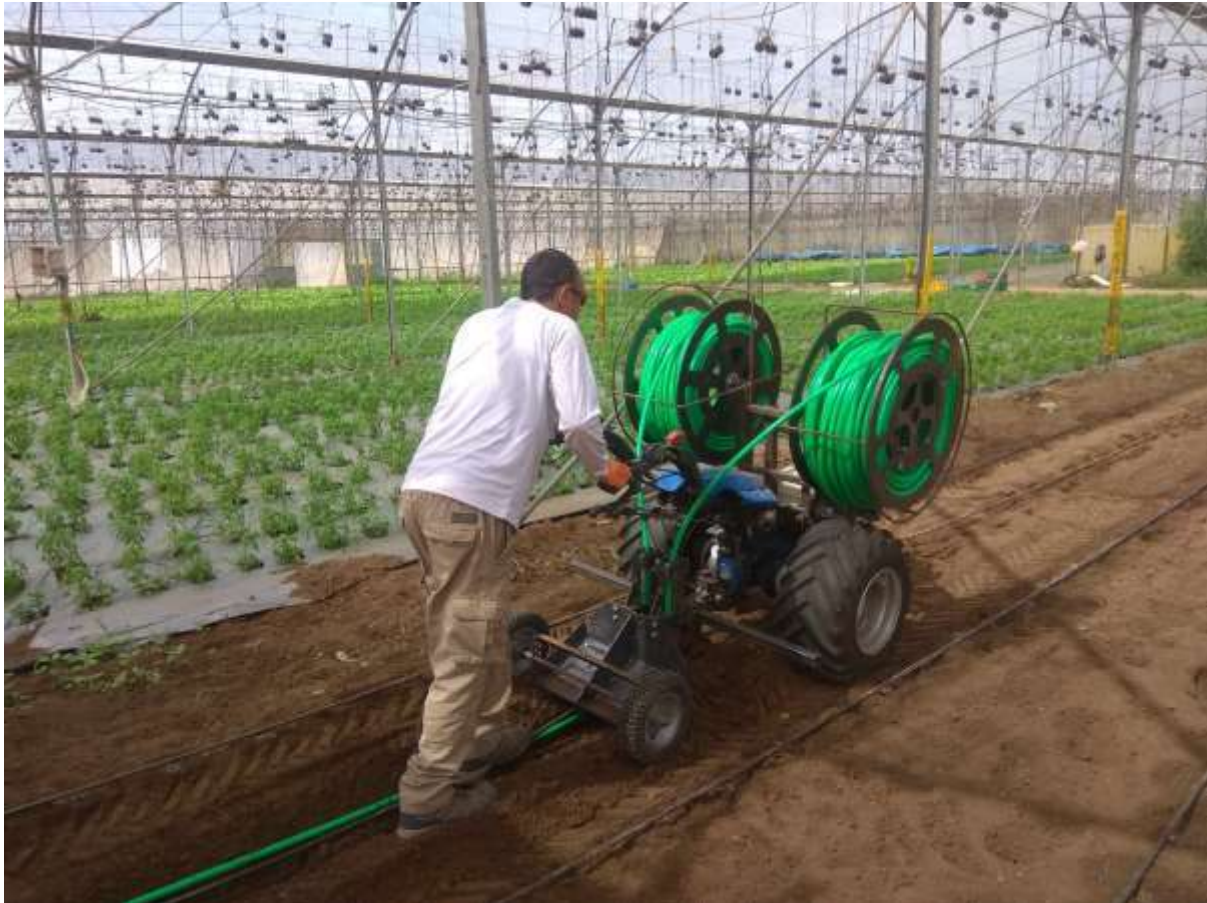
Roots' self-embedding machine being used to install RZTO pipes.
