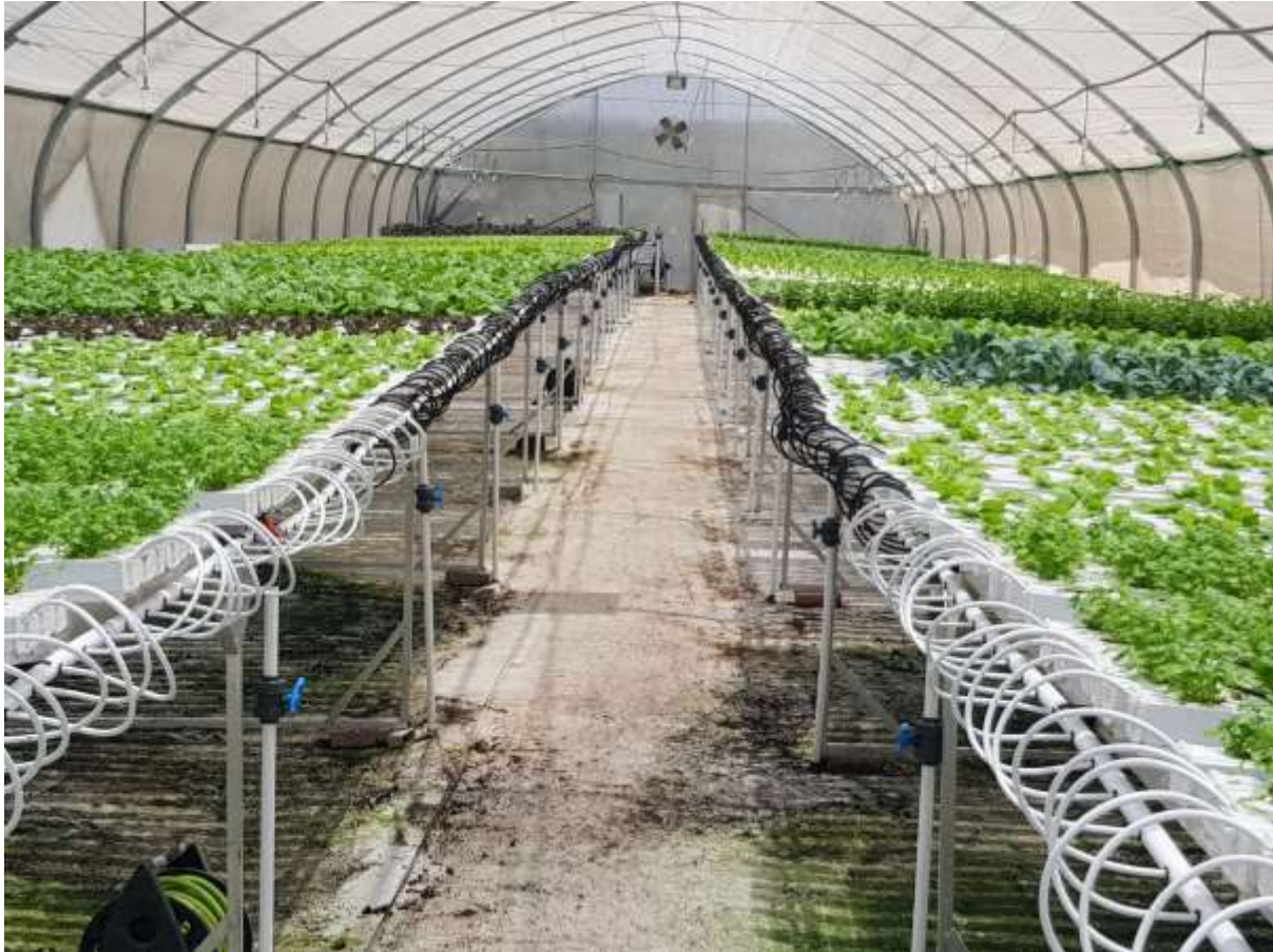
Image: Completed installation at HYDRO GROW hydroponic greenhouse
