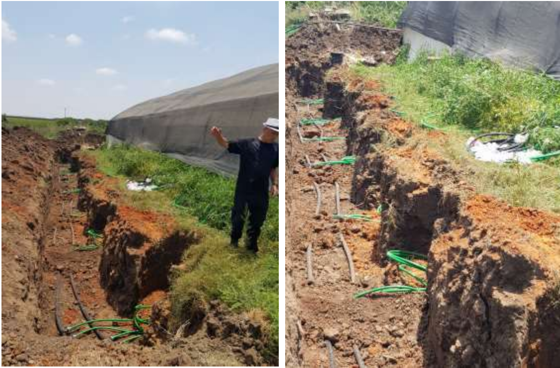
Images: Installation activities at HYDRO GROW
