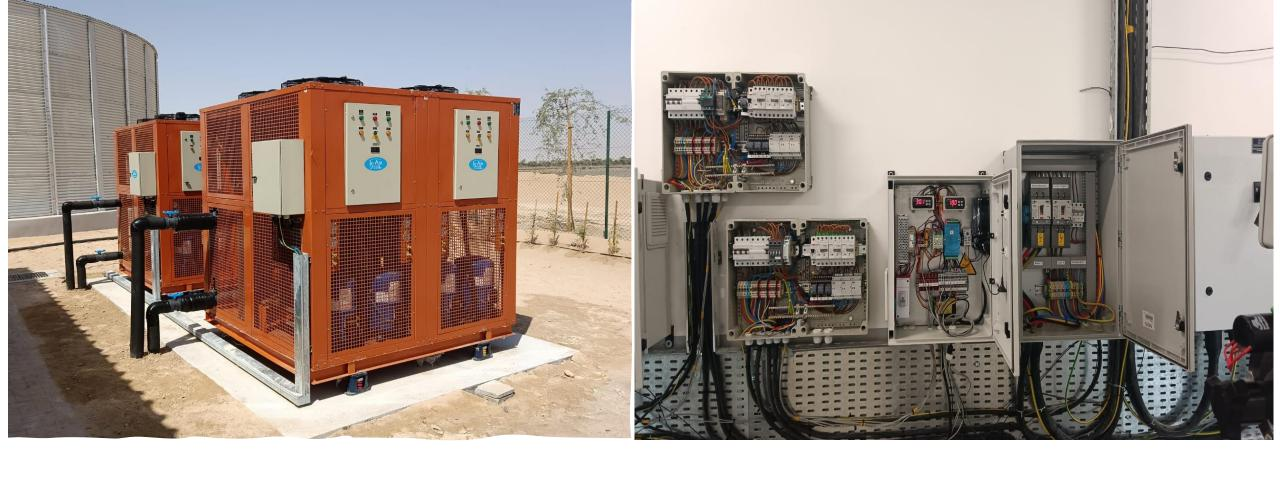
Chillers used for maintaining cooled and optimal root zone temperatures in very hot air temperatures
